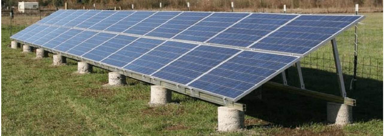
Fixed Tilt Based Module Mounting Structure
